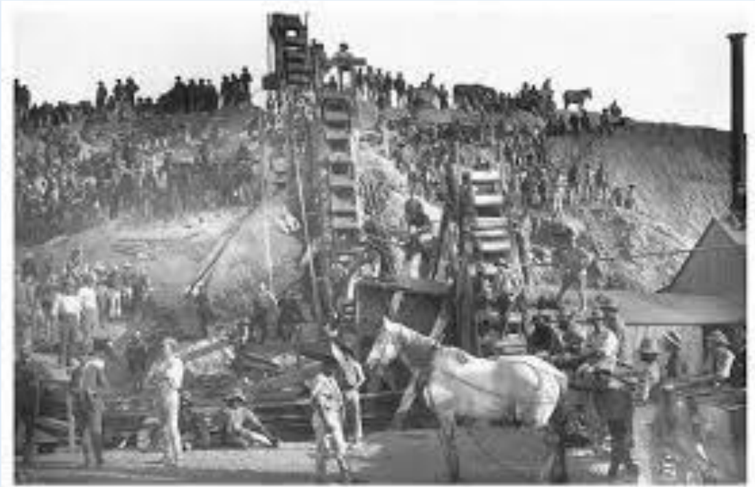
Figure 7: Labourers standing amid machinery for washing diamonds Kimberley, South Africa In this picture above we see what it must have looked like from the outside of the mine:
