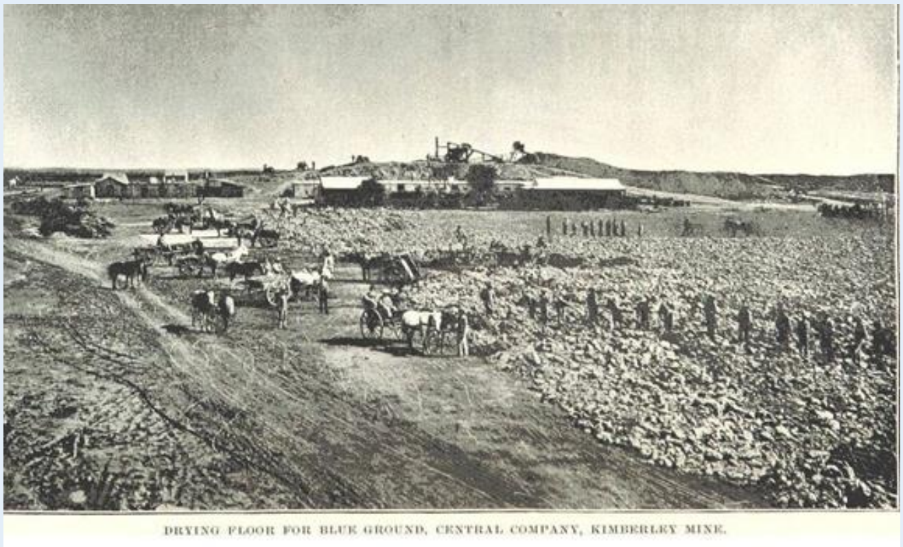
Figure 16: Drying floor for blue ground, Central Company, Kimberley mine
